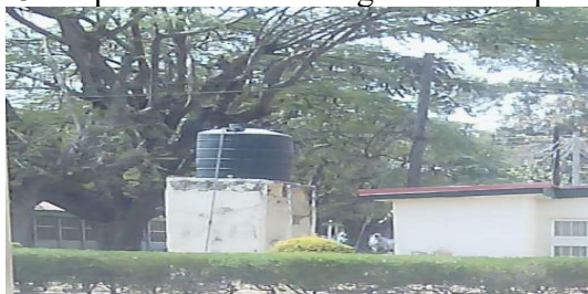
Over Head Water Tank
